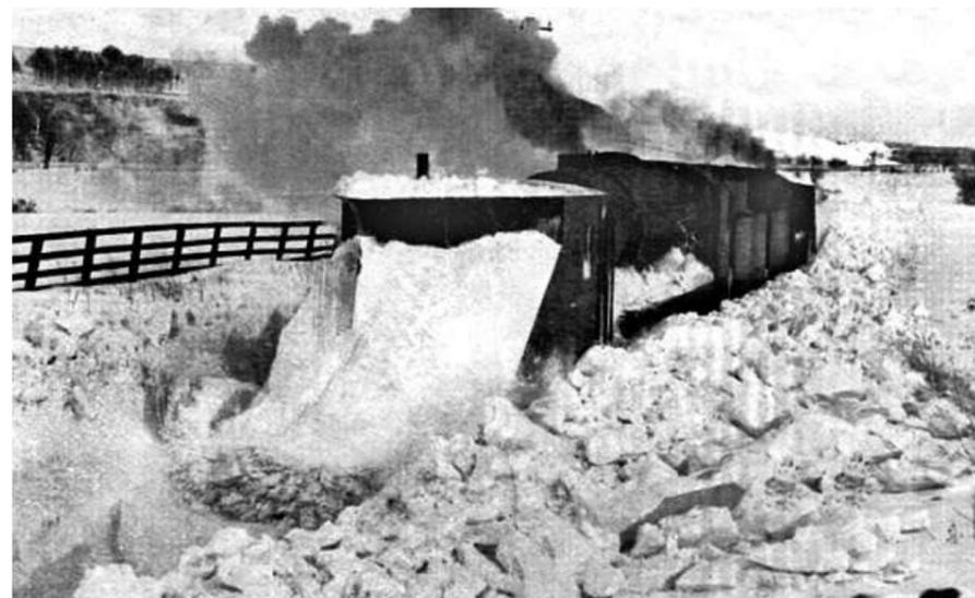
On the second day of snow clearance on the Esk Valley branch Darlington WD's 2-8-0's 90479 and 90593 using North Eastern Railway snowploughs No 18 and 20 clear the line between Battersby and Kildale on 8 February 1963. MAURICE BURNS COLLECTION
